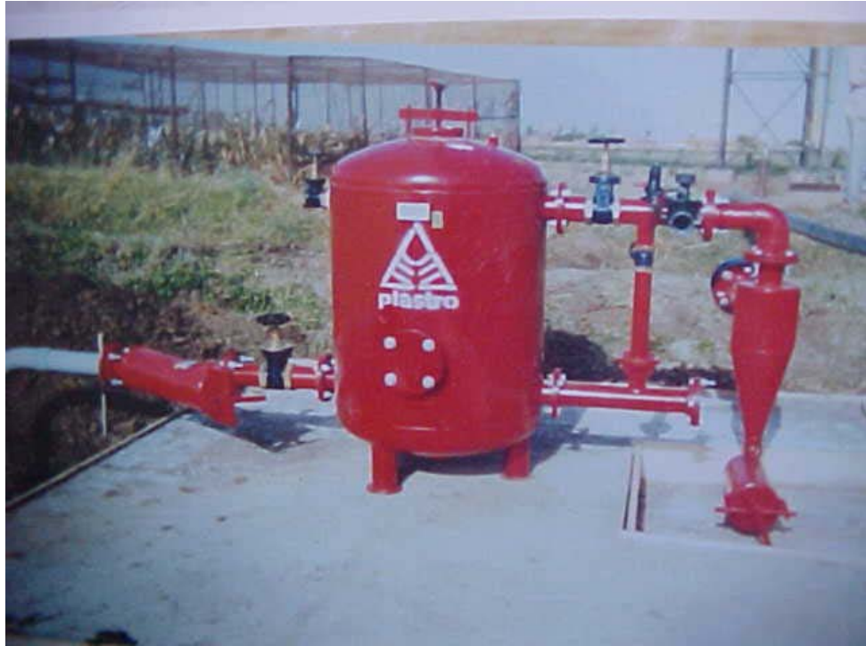
Plate (3.4): The filtration system
